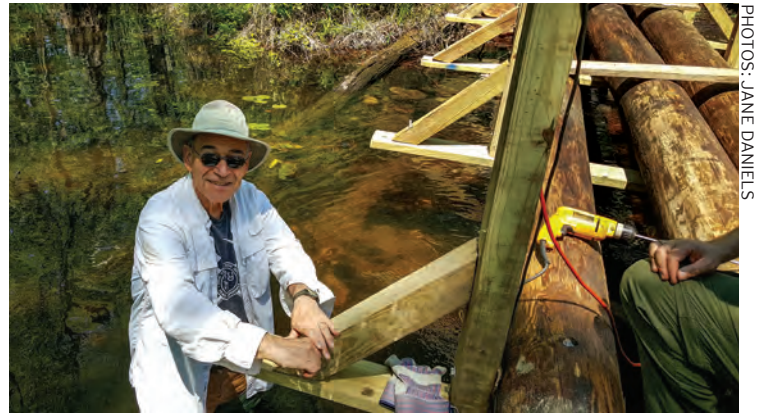
Trail Conference member Bob Gurian worked on the bridge.
